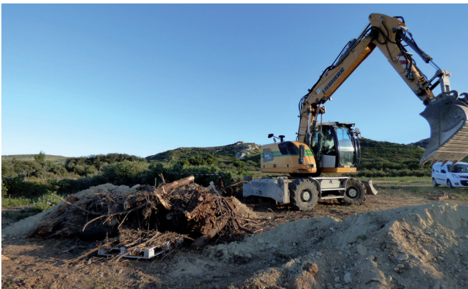
Figure 10 – Construction of rabbit warrens © Alpilles PNR / L. Zechner
